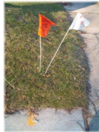
Don't dig with power tools within 18 inches of marked facilities.
